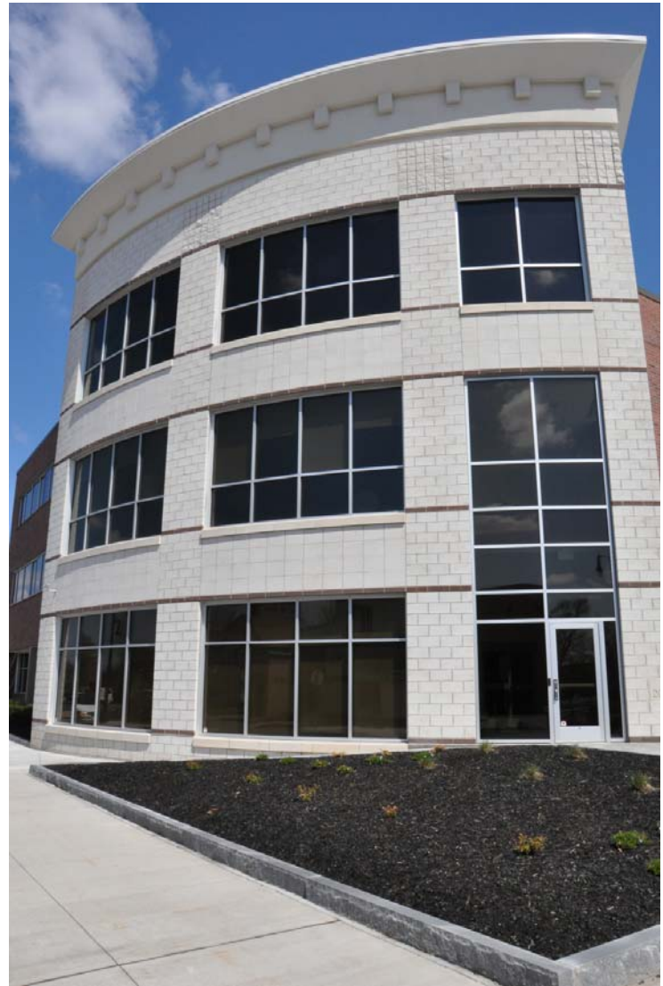
The design of various finishes and sizes of concrete masonry units on a radius gives the façade a monumental scale.
