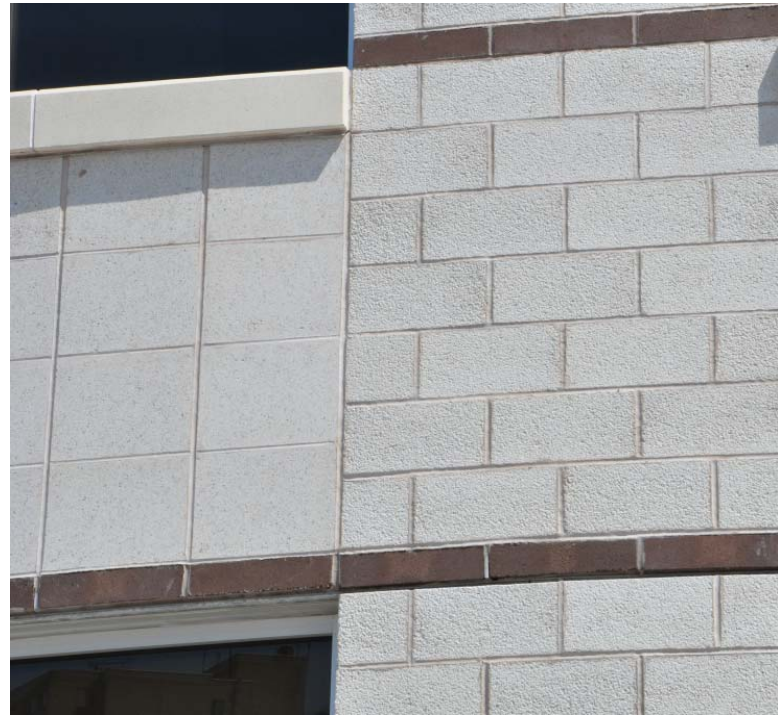
The use of Spec Brik Concrete Masonry Units eliminates Slip Plane Concerns while allowing for a "brick" accent.
