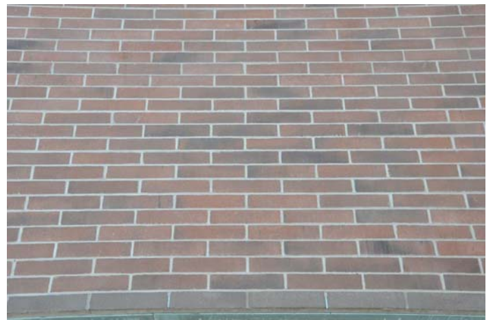
Spec Brick in Running Bond at the Office Addition.
