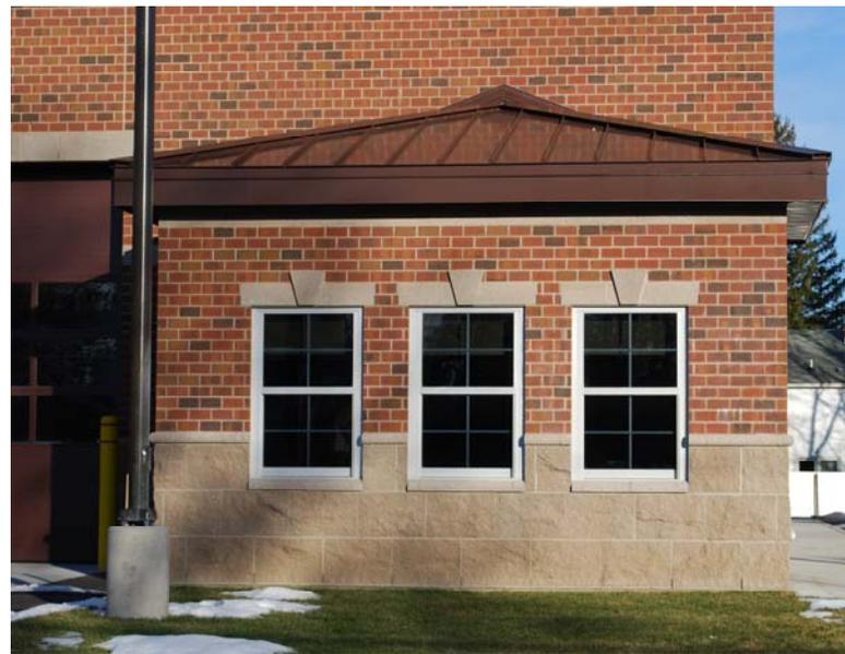
Details such as Keystones, Arches, Sills and Watertables were created using specially fabricated CMU shapes, from large rectangular CMU. The cost of producing these special shapes was a great value and allowed the Architect flexibility in design.
