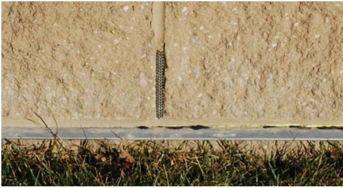
Attention to detail can be seen throughout the project. Flashing and weep details placed at the proper locations to help direct any moisture out of the cavity wall system. A Stainless Steel drip edge is even used to prevent moisture that reaches the flashing from doubling back underneath the flashing at these critical junctions. Control Joints spaced properly and caulked to minimize any potential cracking of the masonry.
