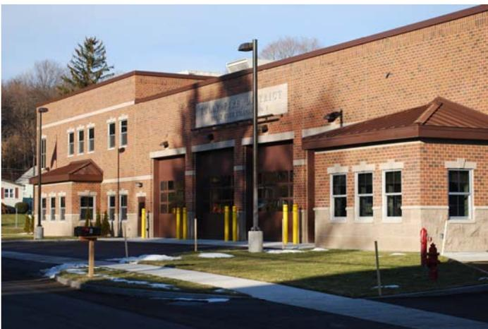
Higher up on the wall, a 4x8x24 Decro Face or Sandblasted course is incorporated into the brick to lend color contrast, but because of its smoother nature, provides a cleaner line in the brick wall.
